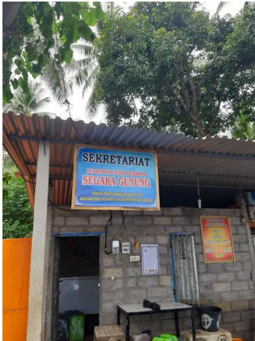
Figure 2.15: The office and fish storage of LFG. Segara Gunung
