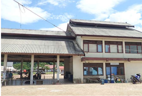
Figure 10.31: The office building of FP Torobulu
