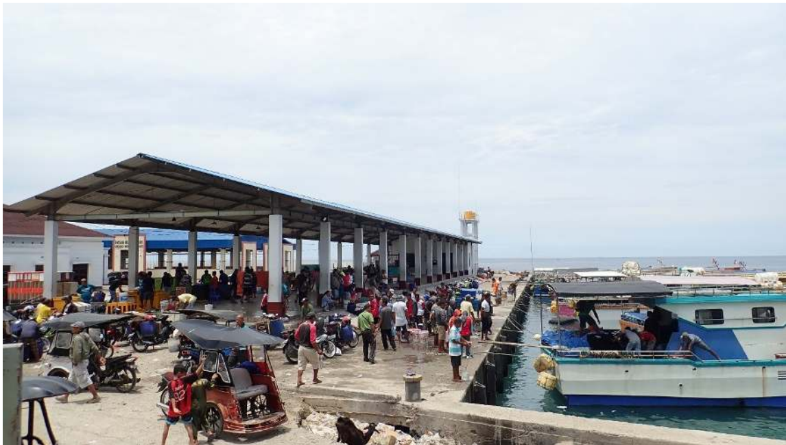
Figure 6.14: One of jetty in FP Inengo
